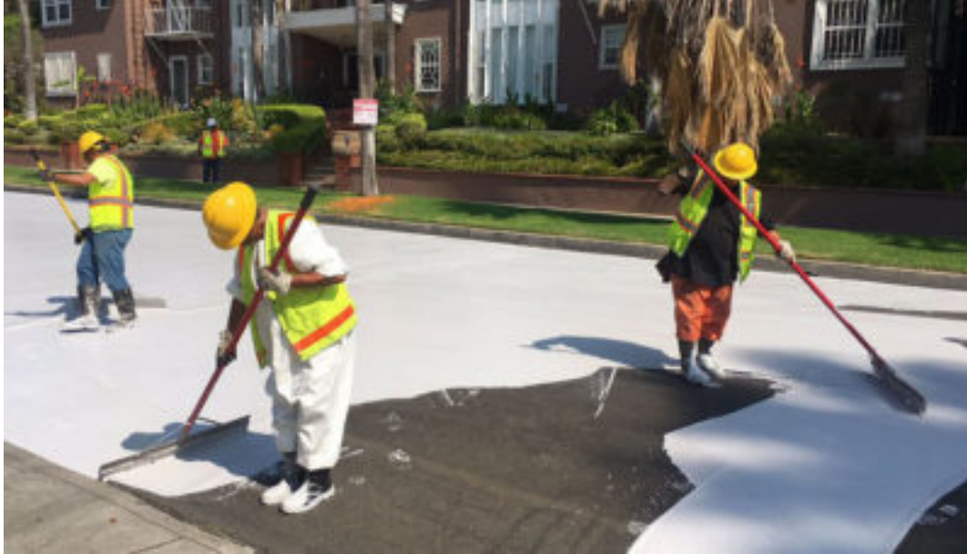
Los Angeles has coated several streets in a light gray paint to reduce road-top temperatures by as much as 10 degrees Fahrenheit. CITY OF LOS ANGELES BUREAU OF STREET SERVICES
