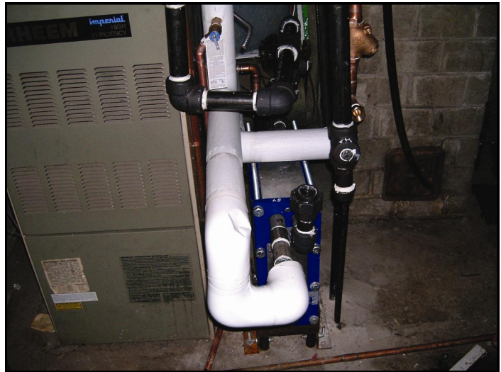
Revelstoke District Heating Heat Exchanger
